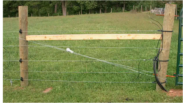
Fig 6. When setting up gates, an ‘H’ brace should be used for correct fence support, and run the charged wire underground to avoid equipment from damaging it.
